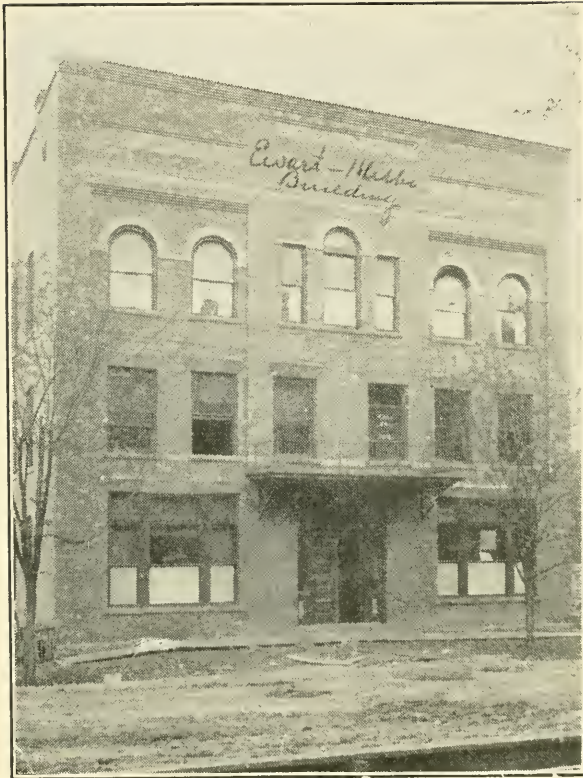
THE EWART-MILLER BUILDING. Erected in 1905.
